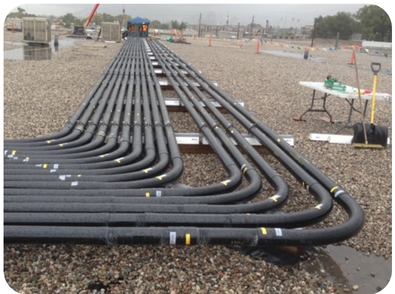
Exposed conduit is subject to environmental factors such as temperature, humidity, precipitation and pollutants that cause corrosion.
