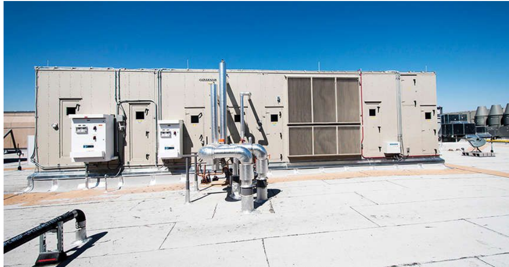
Figure 2: An applied rooftop unit has multiple coils and airside economizer. Courtesy: SmithGroup/Liam Fredrick
