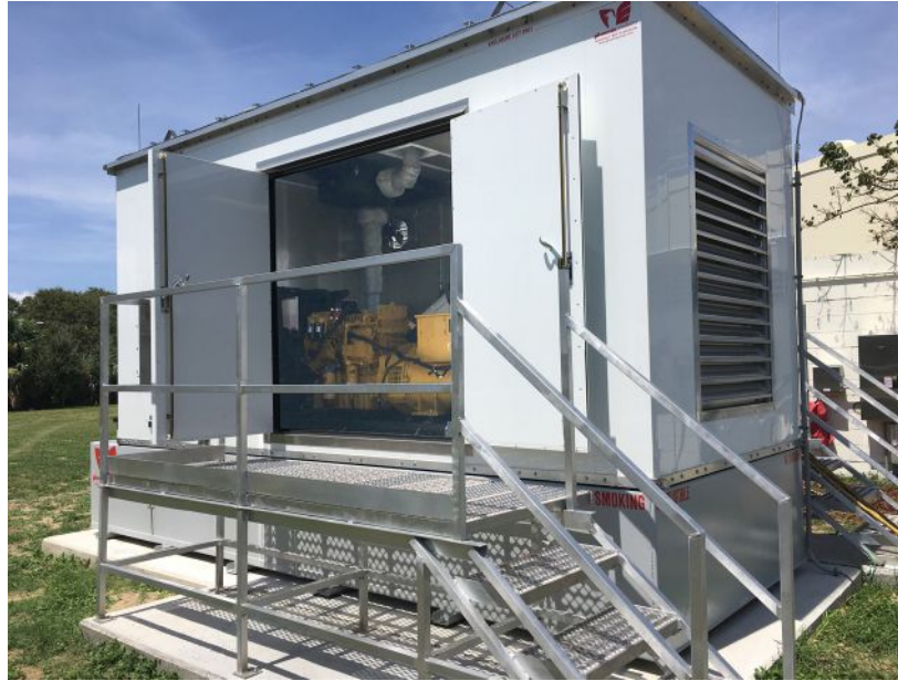
Figure 3: Shown is a generator located in outdoor enclosure with sub-base fuel tank. This image highlights the small site footprint of an outdoor enclosure and the limited amount of space around and within the enclosure for maintenance.
