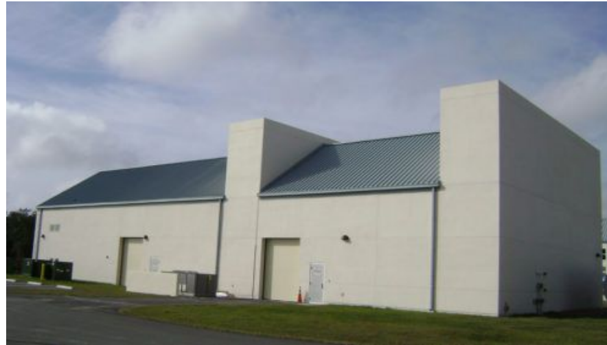
Figure 4: The exterior of an electrical and generator building with intake and exhaust plenums is shown.
