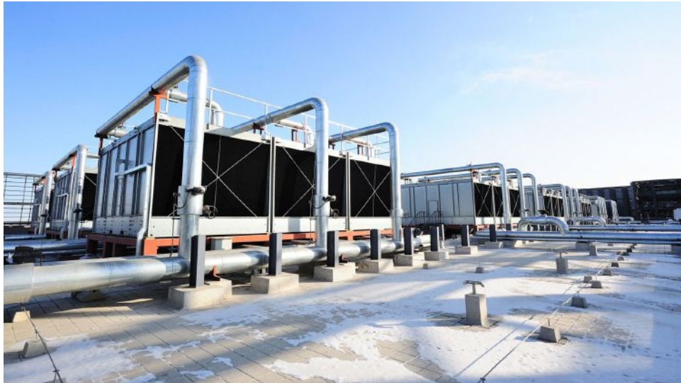
Evaporative cooling towers are an integral part of many data center cooling systems, depending on their location.
