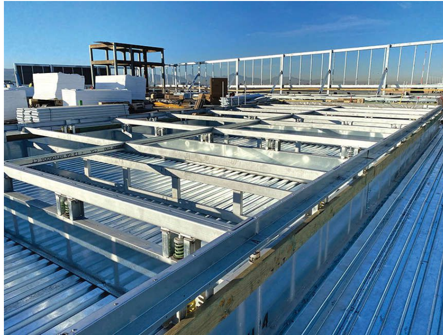
Figure 4: A vibration curb is used to isolate a rooftop unit from transmitting sound and vibrations to the building structure.
